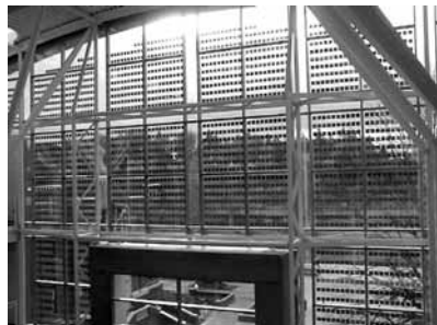
University of Oregon's Lillis building shows PV cells integrated into vertical glass.
