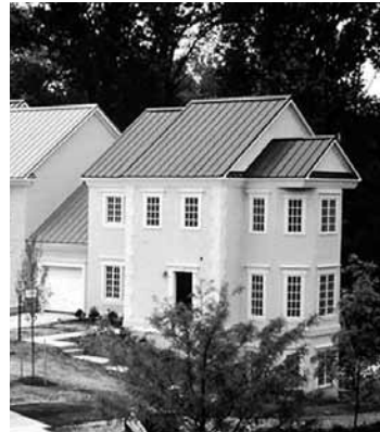
Roof integrated thin-film modules
