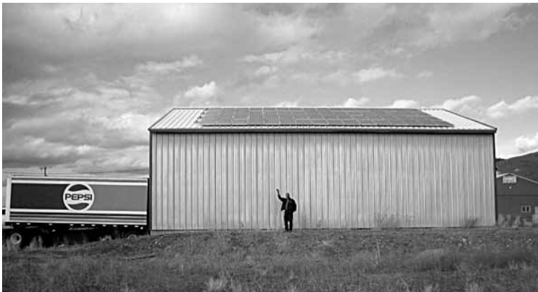
Pepsi's warehouse in Lakeview has a large PV array.
