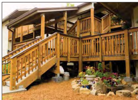
Sandhill Villa in Seaside, a Northwest Oregon Housing Authority development, was built in 1979 with a USDA Rural Development loan. It has 32 units in five buildings.
