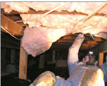
Installing insulation under house.
