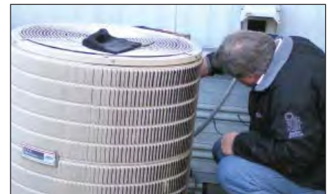
Replacing a heat pump for a mobile home resident.
